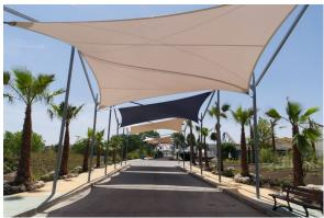
Tensioned textile covers supported by cables or perimeter posts that are designed to maintain the membrane under tension, complemented by a sturdy metal structure to withstand external forces. Customizable designs can be tailored to fit the available space, offering options for one or two slopes, as well as vertical enclosures on the sides and/or rear, depending on the specific requirements.
